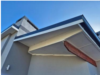
Pic 01: Patio balcony roof construction.
