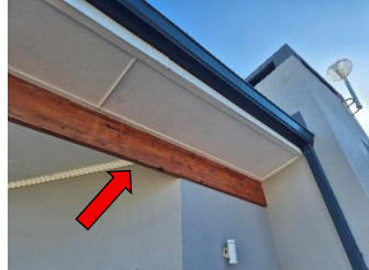
Pic 02: Timber beam in support of roof structure.
