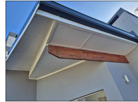
Existing configuration of Patio Roof supported by Timber beam
