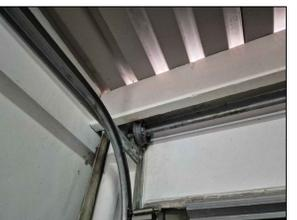
3. Rainwater seeping from internal gutter.
