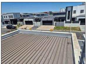
2. Damaged roof sheeting and wall flashing.
