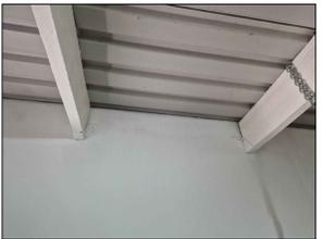
8. Wooden rafters fixed to wall with low spec bracket.
