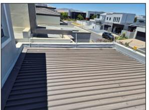
1. Loose wall flashing and deflected roof sheeting.
