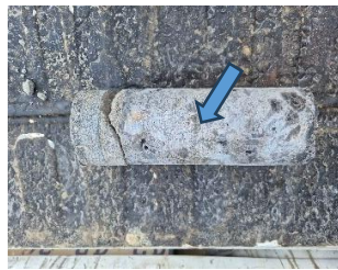
Pic 20: Core #01 with air-pockets, result of poor vibration.
