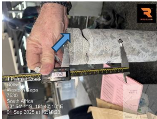
Pic 19: Core #01 measure rebar 125mm from top.
