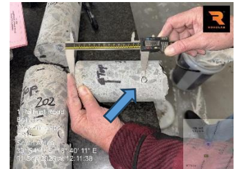
Pic 22: Core #03 – rebar located 134mm from top of slab.
