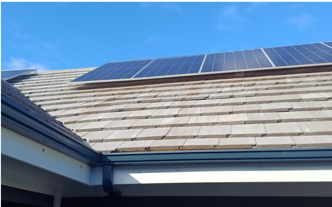
Figure 3: Tile installation not neat some tiles lifting.
