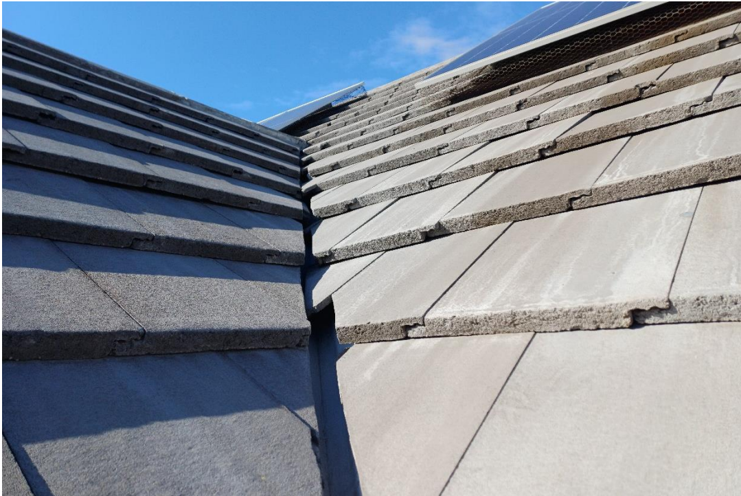
Figure 2: Roof tiles loose and slide out of position over valley gutter.
