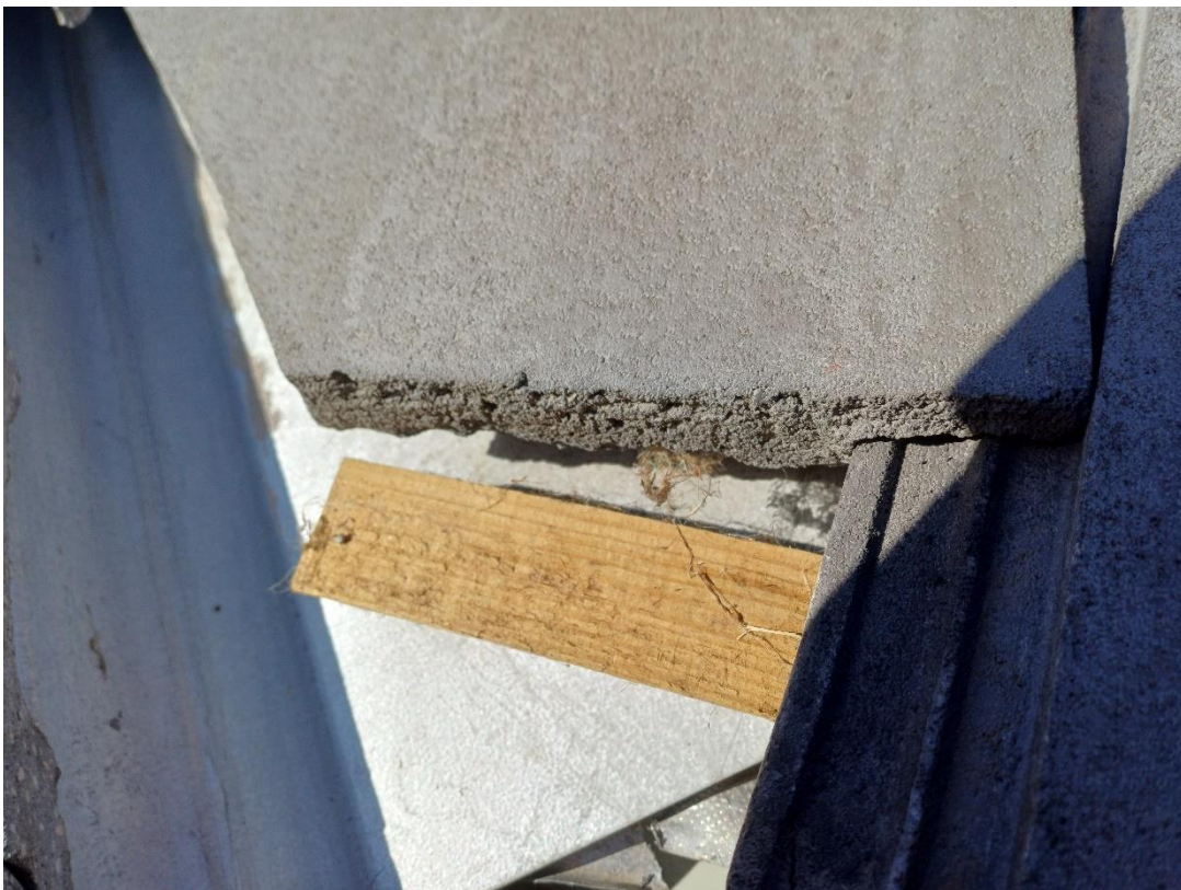
Figure 5: Loose tile pushed back exposing the batten.
