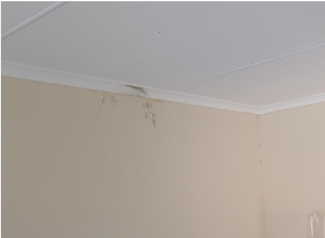
Figure 6: Water damage on the northwestern garage wall at the cornice.
