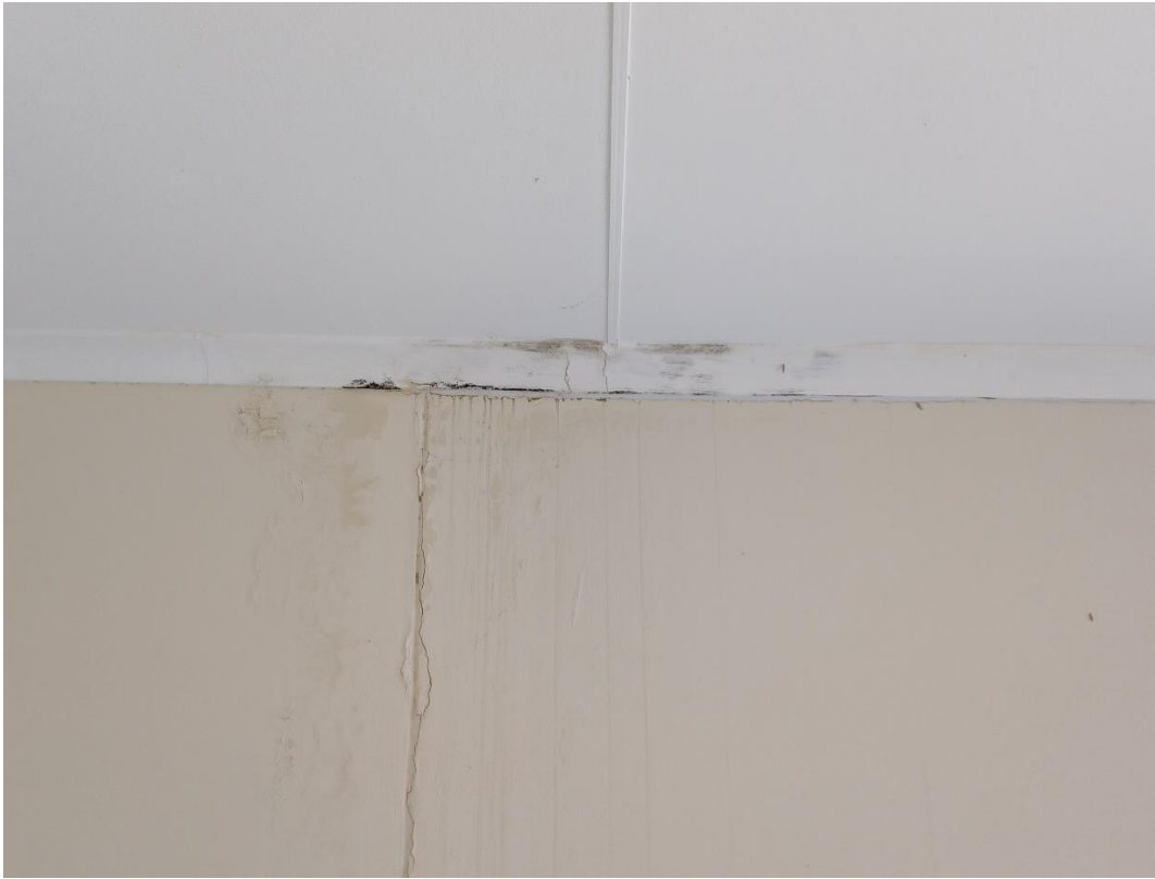
Figure 5: Water damage at control joint on southeastern wall of garage.
