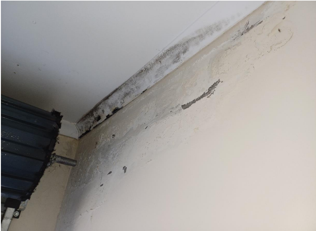
Figure 3: Damp damage at the western corner of the garage.
