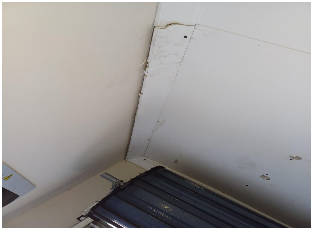
Figure 4: Water damage on cornice in southern corner of garage
