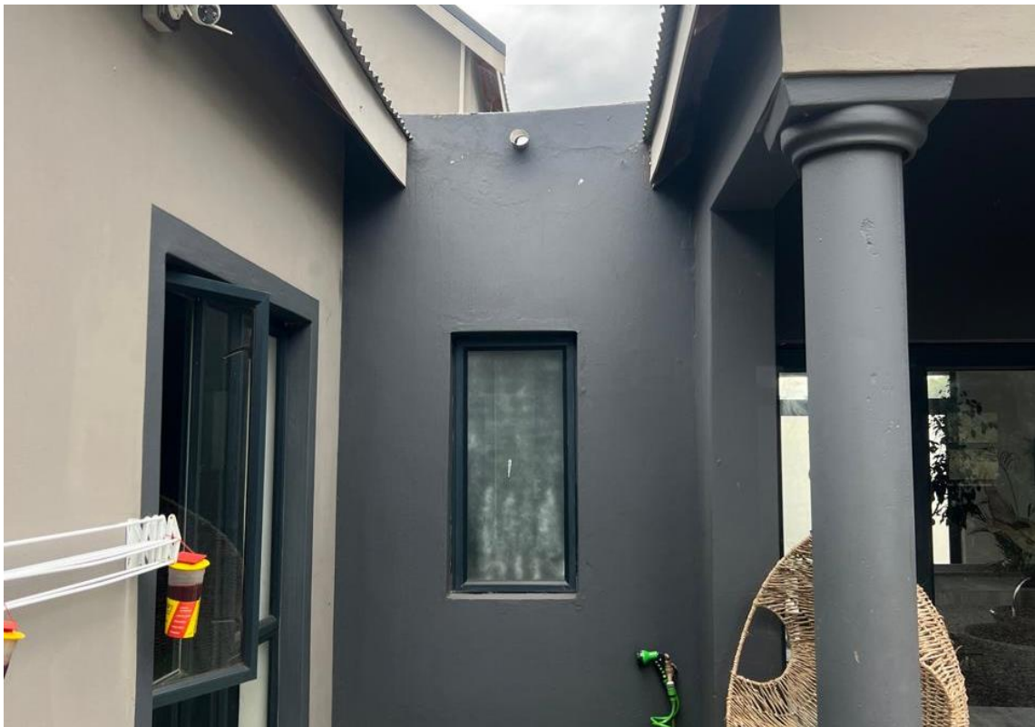
Figure 3: Front elevation with horizontal parapet wall crack
