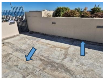
Pic 06: Damaged construction joints and waterproof edges.
