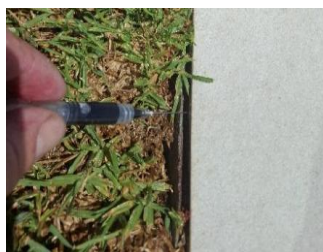
Pic 02: Waterproofing of grassed area next to pool peeling off.
