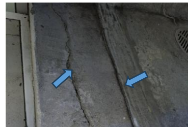
Pic 07: Cracks in concrete slab above house entrance on 2 nd Floor.
