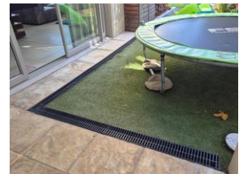
Pic 04: Artificial lawn lower than water channel.
