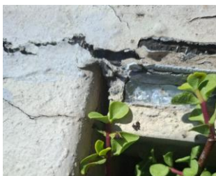
Pic 01: Damaged waterproofing at corner of Plant Box.
