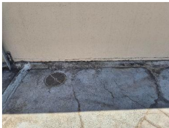
Pic 05: Full-bore level with surface and visible cracked concrete surface.
