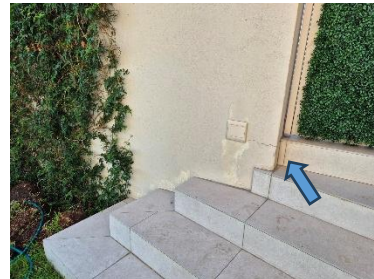
Pic 10: Rainwater from the adjacent stairwell entering the property.
