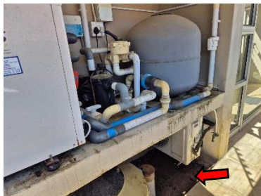
Pic 08: No concrete surface below HVAC equipment on Ground Floor.
