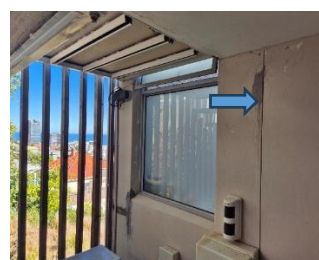
Pic 13: Structural cracks at movement joints.
