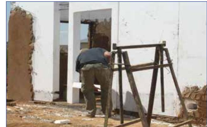
II ▶ EPS Bygg external walls covered with mesh and plaster
