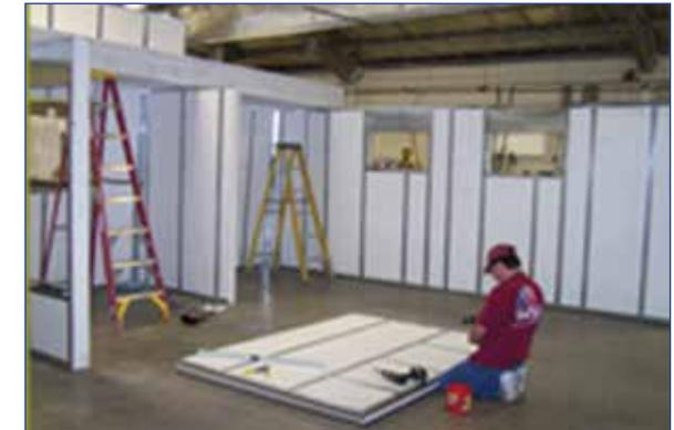
II ▶ Ecodwell panel walls showing EPS core and lightweight steel framing
