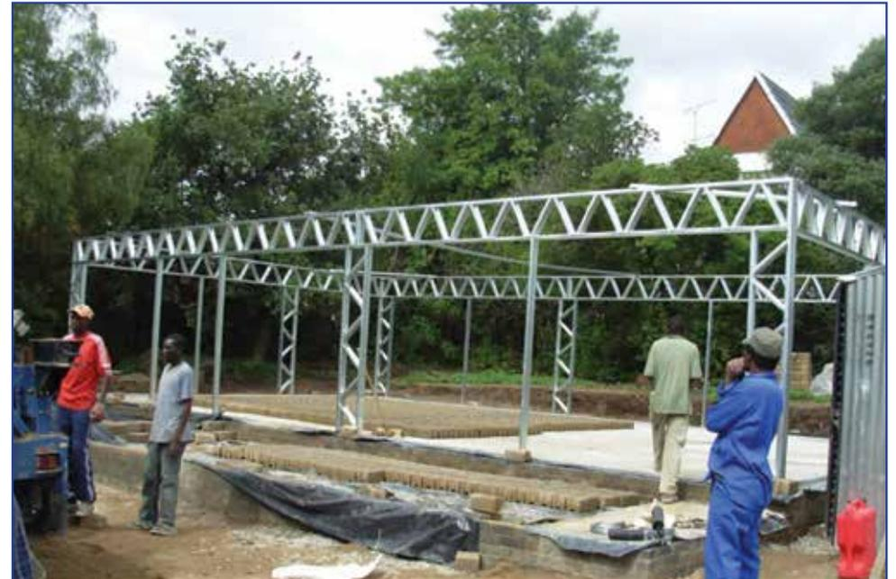
Powerwall main lightweight steel frame
