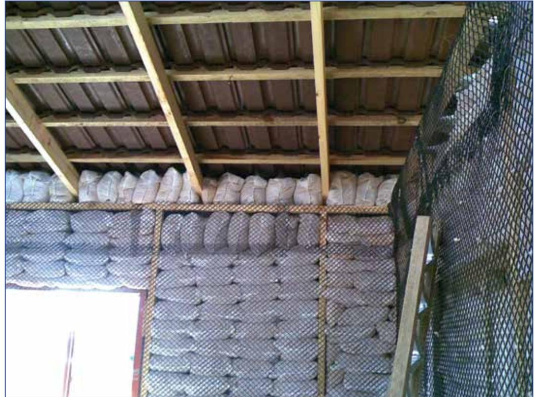
III Eco-beam external wall and sandbag infills
