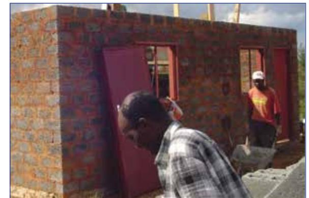
II ▶ Intercon external wall using Polycon cement block
